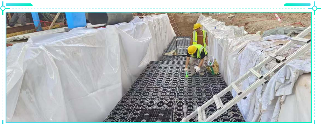
The PP modular water storage tanks adopted by the Appotronics Headquarters Tower project
