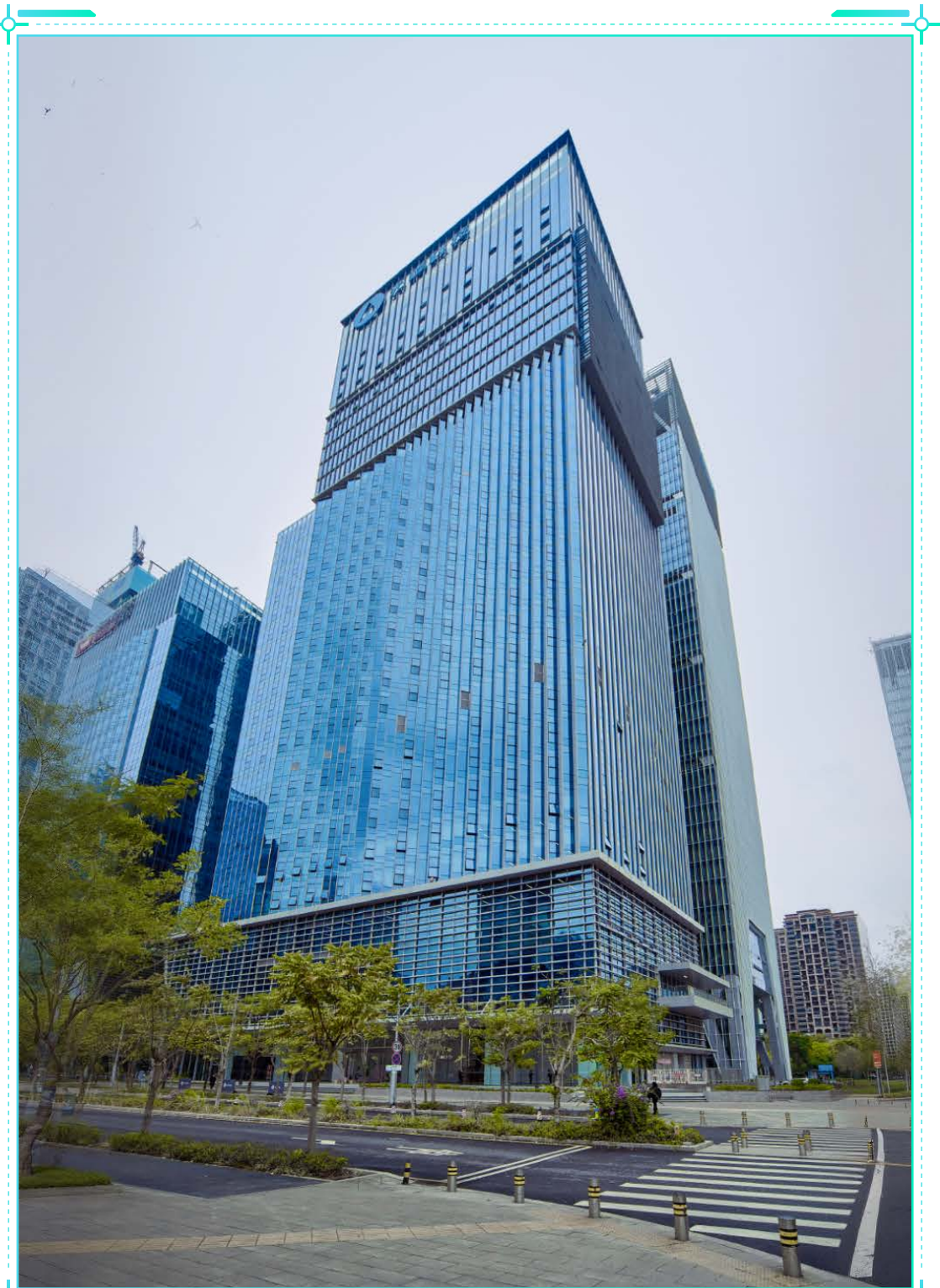
Overall view of Appotronics Headquarters Tower
